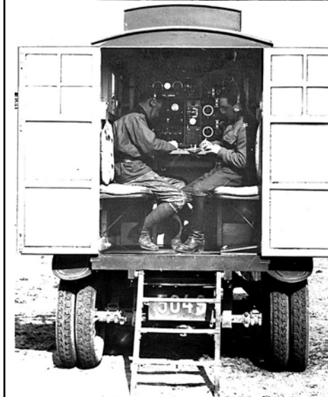
Signallers in a Renault MH2 vehicle operating a RKG/A with original Marconi YC3 receiver.
